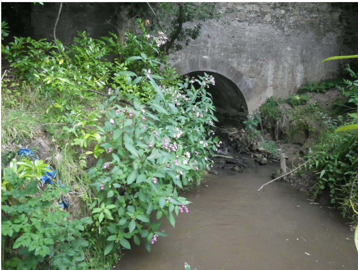
Plate 6. Himalayan balsam on Edermine stream downstream of Glebe Bridge.
